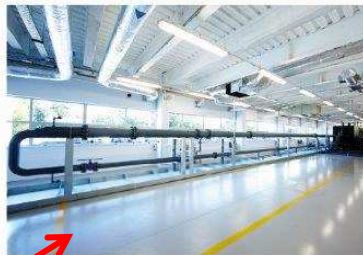
Large Multi Phase Flow Loop (LMPFL)
